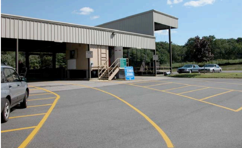
In front of the transfer station operator's booth
